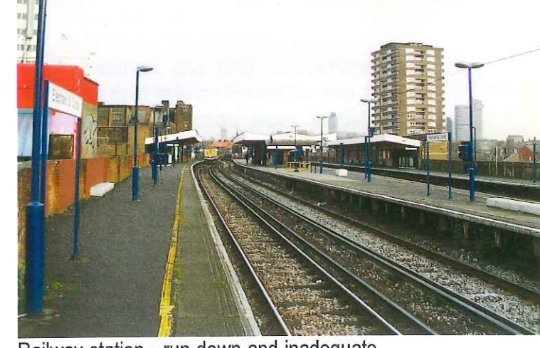
Railway station - run down and inadequate
