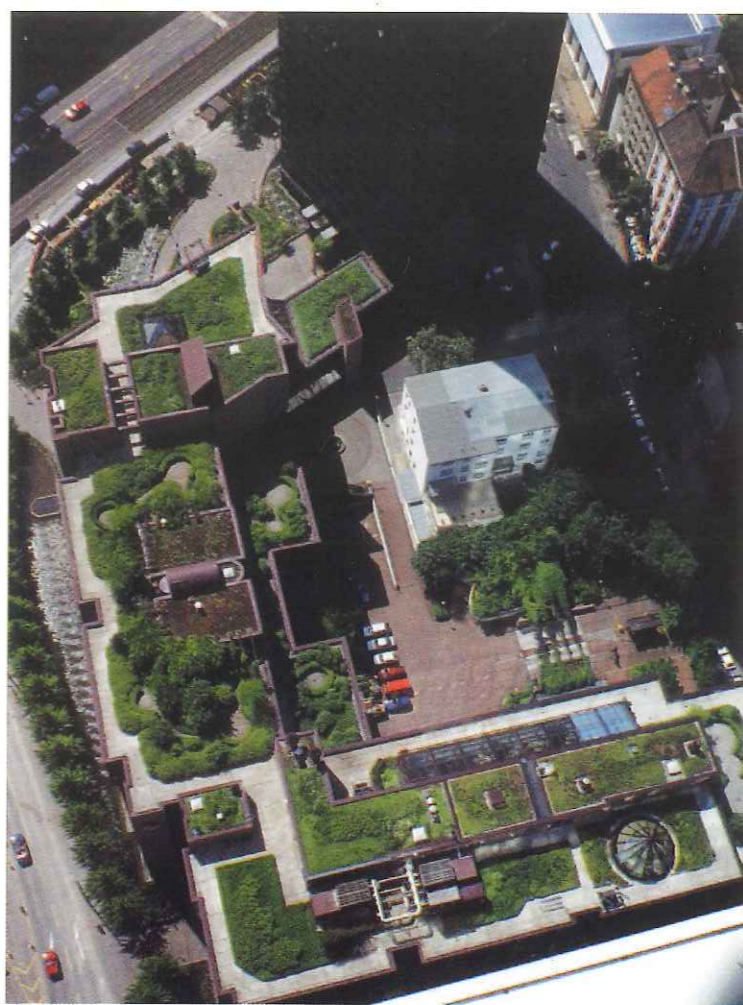
Organic rooftop gardens
