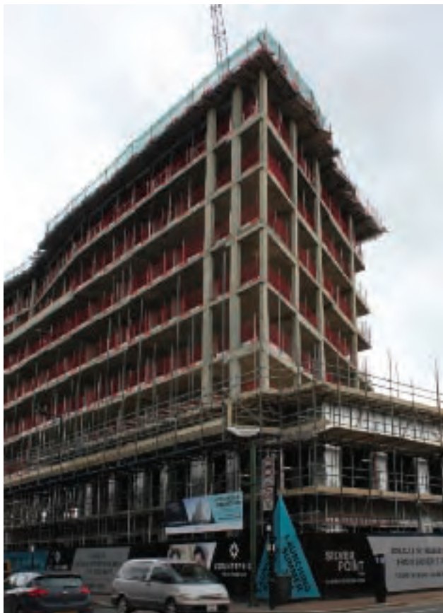
Building under construction
